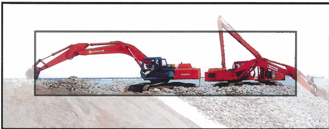
construction in progress : March 2004
