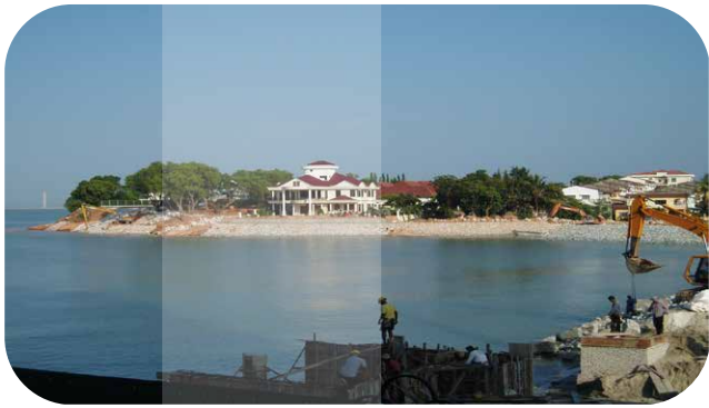
Reclamation works are approaching completion with protective rockbund in place.
